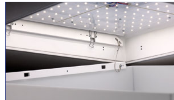
BELOW CEILING ACCESS
