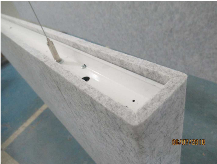
Figure 2 - Detail of individual baffle
