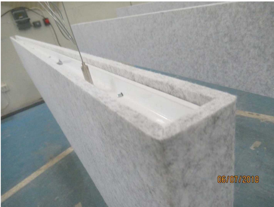
Figure 2 - Detail of individual baffle
