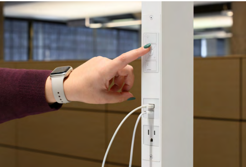
User conveniences include local dimming controls, USB-A/USB-C & 120-volt charging ports.
