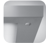
daylight / occupancy sensor
