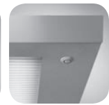
daylight / occupancy sensor
