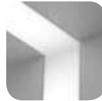
wall to ceiling corner
